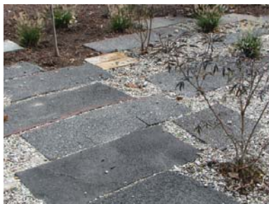
Hand cut/hand set recycled asphalt pavers
