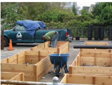
Groundwork Garden Community Garden, Building raised beds on asphalt
