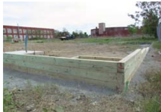
Corner of finished wall with corner dead-man
