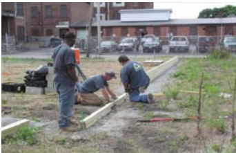
Installation of 16.5" timber wall at 6 degree angle
