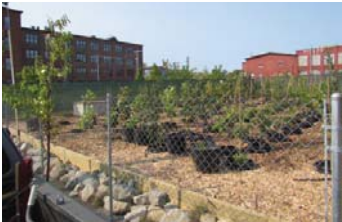
Fence installation, windscreen installation and tree installation
