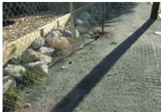
Finished installation of Geo-Block™ permeable sidewalk
