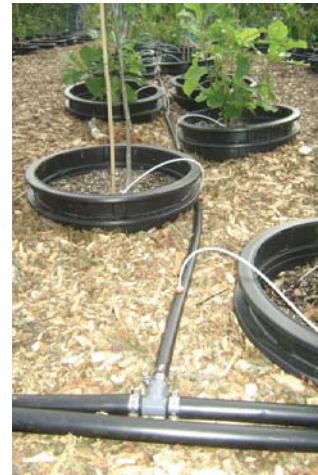
Installation of spray irrigation system
