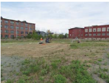
Initial survey, site grading and first course for retaining wall
